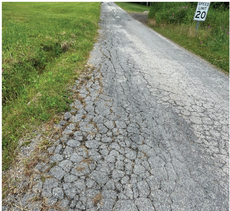
Figure 3-6: Snells Hill High Severity Alligator Cracking
