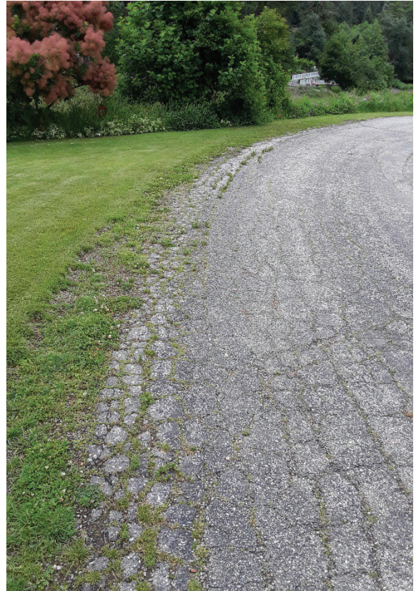
Figure 3-3: Main St. Alligator Cracking
