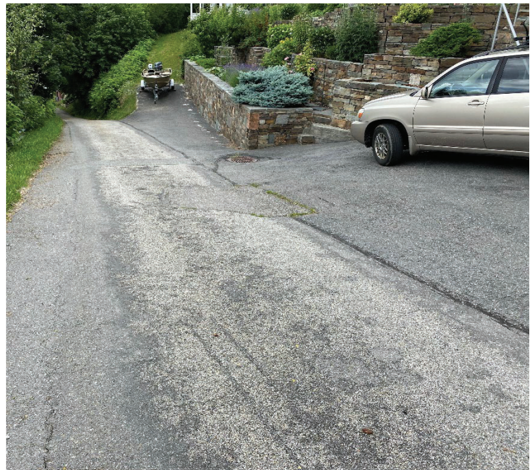
Figure 3-8: Aspen Ln. (Patching, Aging and Raveling)
