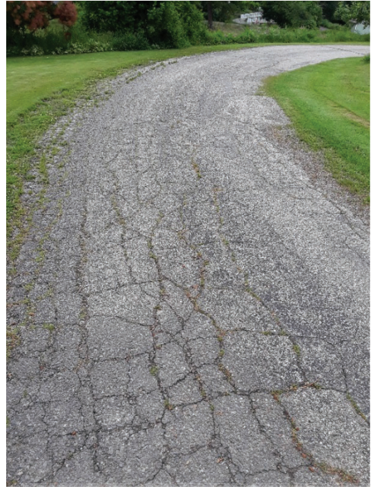
Figure 3-7: Main St. (Northern Section) High Severity Alligator Cracking
