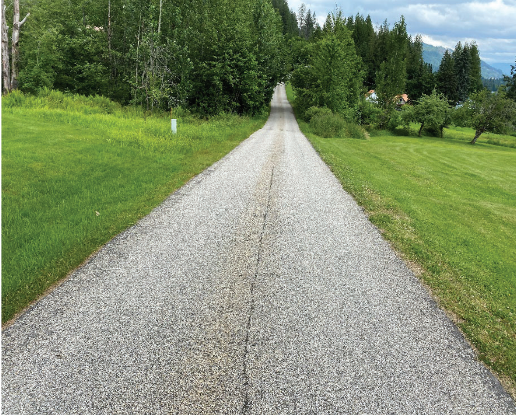
Figure 3-4: Spring St. Longitudinal Cracking
