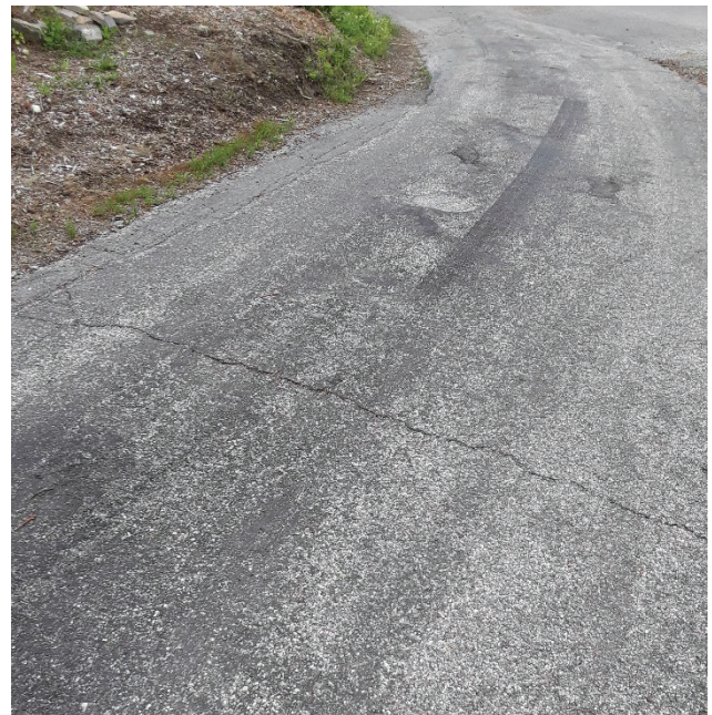
Figure 3-5: Main St. Transverse Cracking
